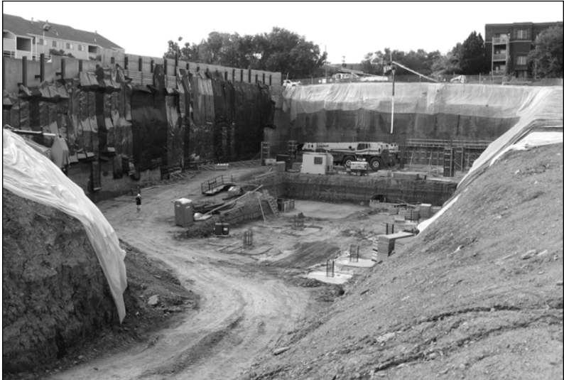
Excavation of the Oread Inn site - Underground Parking There will be four levels below grade that will accommodate; 200 off-street parking spaces and a “basement” space that will provide access to commercial space from Indiana and other spaces associated with the hotel such as the theater.
